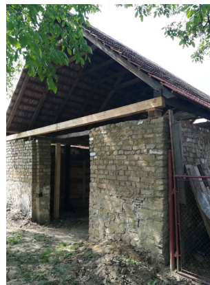
Example of vernacular architecture in Southern Moravia, where earth was used as a building material – barns in Hrubá Vrbka photo: Eva Neumayerová
