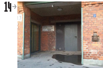
The entrance to Speicher XI in Nov. 2017 Authors' own photo
