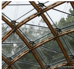
Gridshell structure over the orangery in Chiddingstone, England, detailed view
