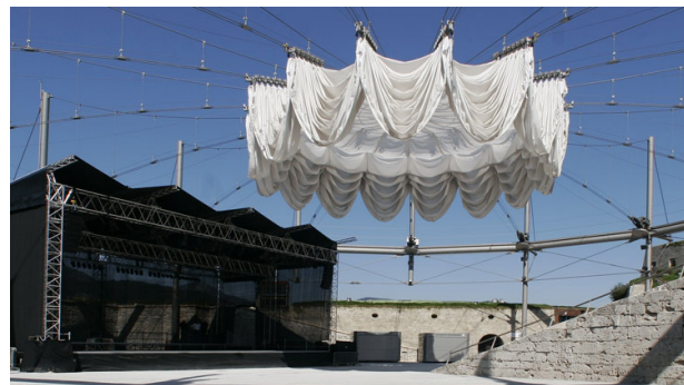
Kufstein fortress retractable roof, Austria, opened situation [3]
