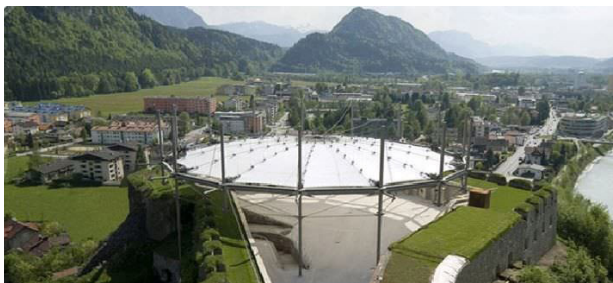
Kufstein fortress retractable roof, Austria, closed situation [3]
