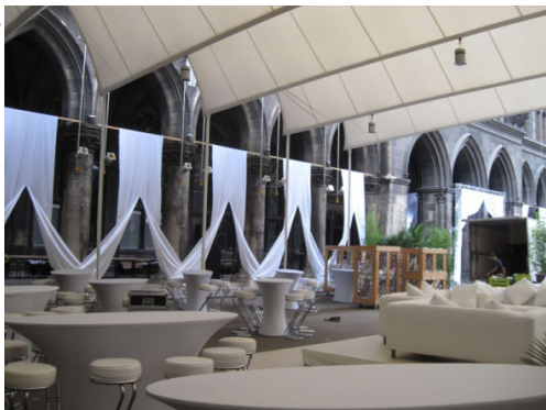
The retractable membrane roof, Vienna town hall courtyard, bird view Formfinder database https://www.formfinder.at (15.8.2018)
