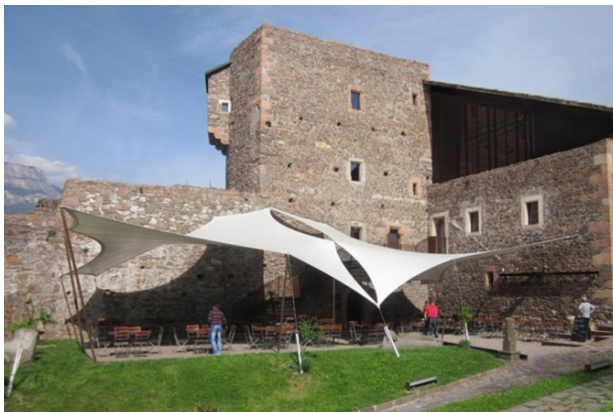
Shading canopy over a restaurant terrace, exterior view [2]
