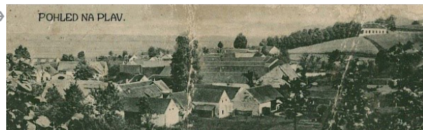
An example of a typical arrangement of village buildings (Plav, okr. Č. Budějovice, about 1920)
