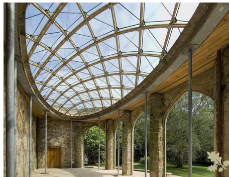
Gridshell structure over the orangery in Chiddingstone, England, interior view
