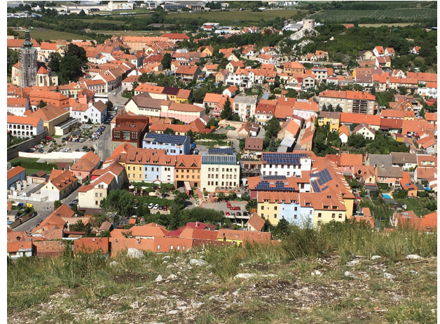
A deterrent example of photovoltaics use—insensitive roof-mounted PV installations on residential block in the urban conservation area of Mikulov, Czech Republic.
