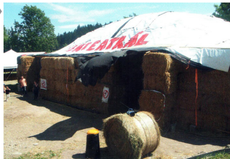
Gridshell roof over the Menteatrál theatre in Neratov, exterior view POLÁČEK V., POKORNÝ V., Recycled Theatre, Praha: Grada Publishing a.s., 2015, page 309-310, ISBN: 978-80-247-5751-3
