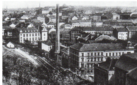
View of the Žižkov power station chimney, the power plant hall visible only partially and just behind the chimney
