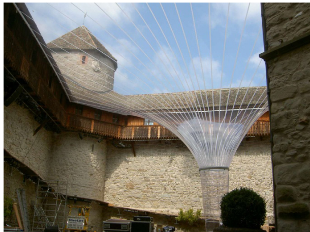
Rain protection canopy over the castle courtyard, exterior view
