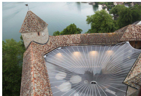
Rain protection canopy over the castle courtyard, interior view
